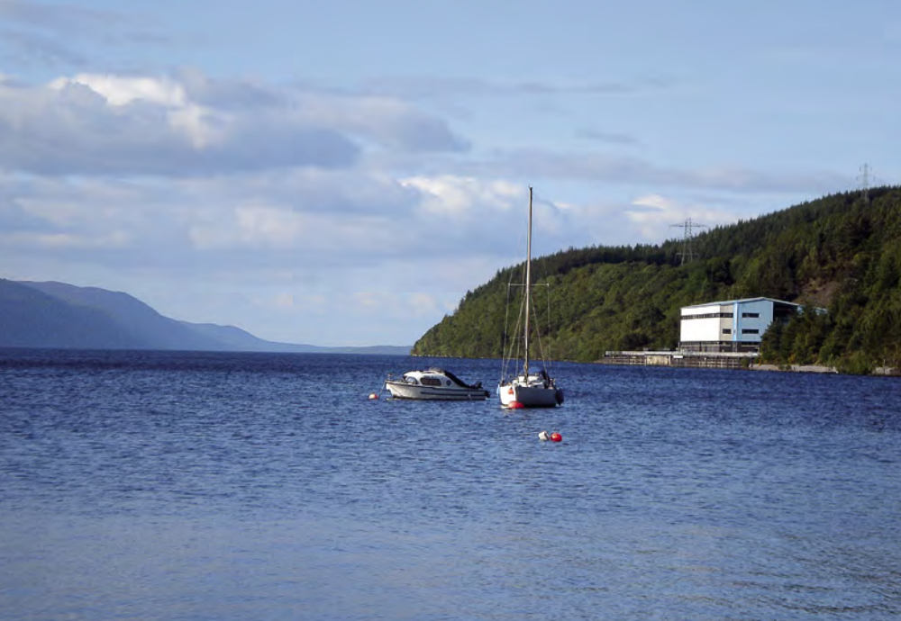
Located by the idyllic Loch Ness, Foyers' pumped storage plant is key to Scotland's grid stability. Voith's regular monitoring and maintenance secure its accurate operation.
