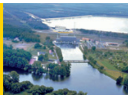
Dychów hydro power station.
