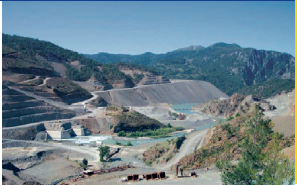
Akköprü construction site.
