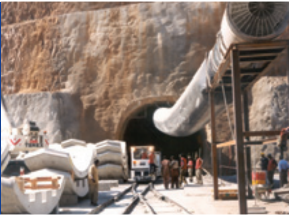
Outside the tunnel of Gilgel Gibe II.
