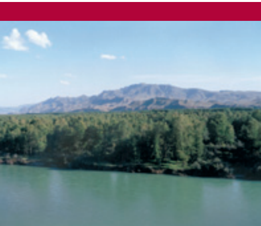
Outside view, Jilintai, China.
