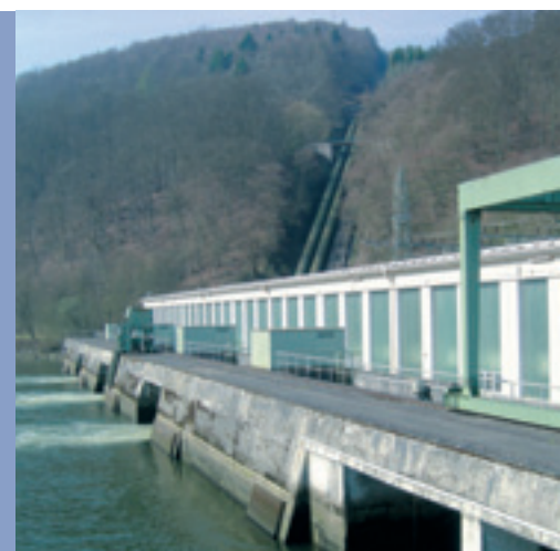
Waldeck hydro power station.
