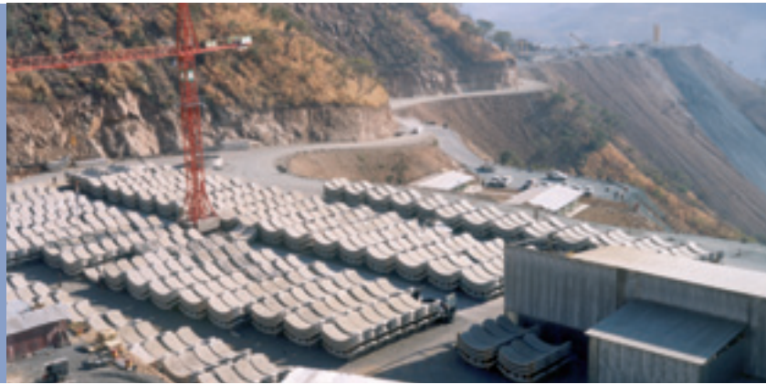
Parts of tunnel before mounting.
