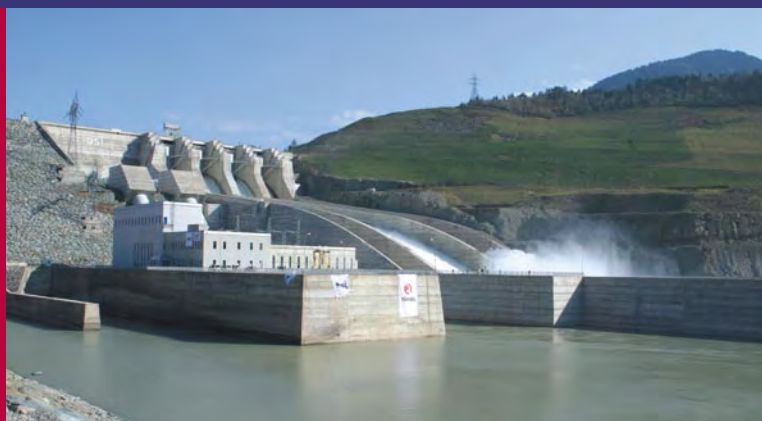
Hydro power plant Borçka on the Çoruh River in northern Turkey.
