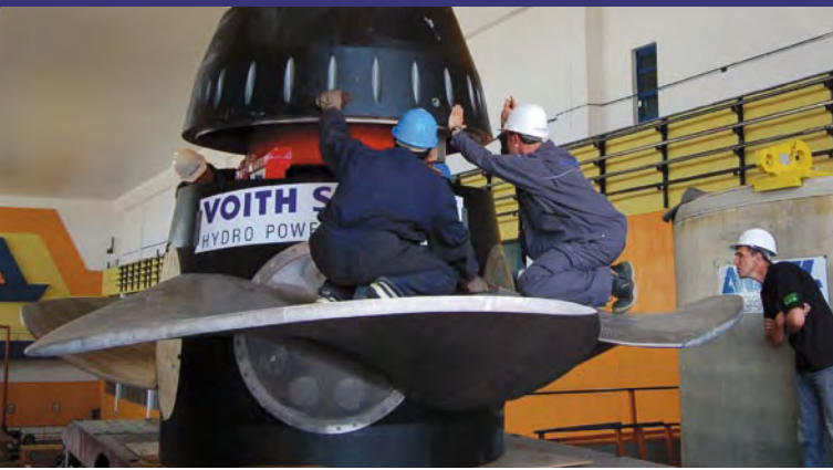
Dismantling of the runner hood.
