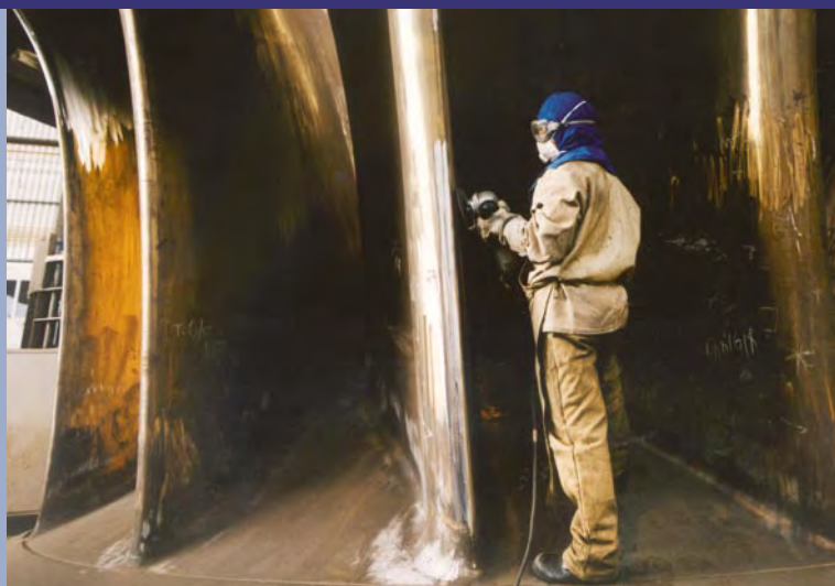
Work on a Francis runner.
