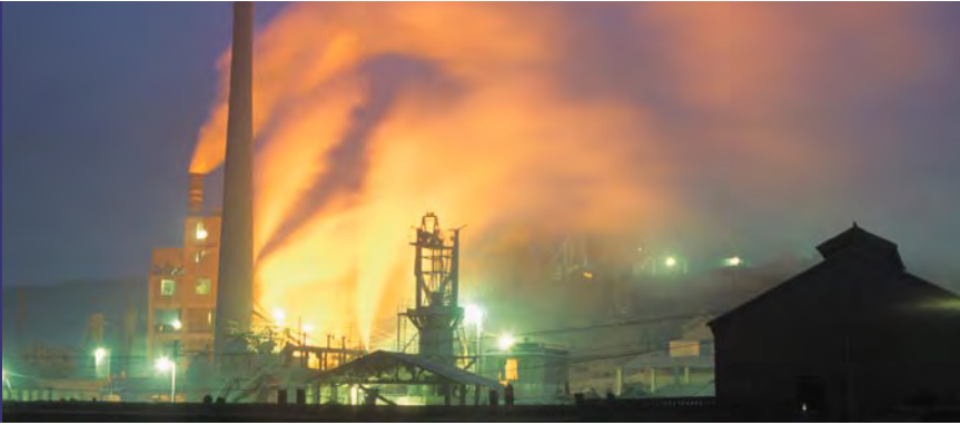
A power station at the site of the Yellow River diversion project in Shanxi province.
