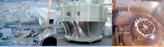
Borçka power house on Coruh River. Borçka: Runner in final phases of manufacture. Borçka: Pre-assembly of unit 2 spiral case and finishing of unit 1 spiral case for site pressure test.
