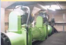
Micro tubular turbine installed on Egasaki Drinking Water Treatment Plant (Serial arrangement of 2 units). Hydro power resources can be harnessed not only from natural bodies of water and developed reservoirs: factories, waterworks, sewage treatment plants and irrigation canals also hold an enormous potential. Non-utilized head as a byproduct of line operation could be employed very effectively for on-site power generation. Application range of micro tubular turbine.
