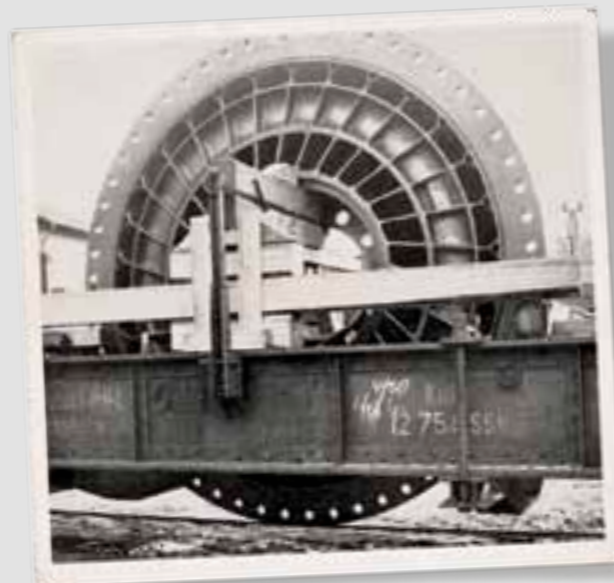
The primary blade wheel (pump) of the start-up coupling for Herdecke pumped storage power plant.
