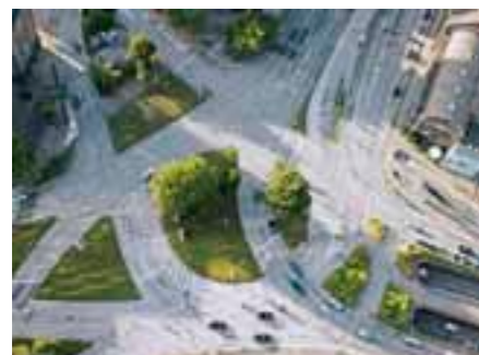
View to the Deichtor Square: Hamburg's road network is continuously optimized.
