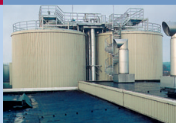
Fig. 8: The new MC stock storage towers.
